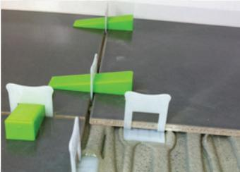
Set the adjacent tile firmly into the adhesive. Butt the tile against the LEV TEC clip giving the 1.5mm joint (if a larger joint is required spacers can be used, or set the required joint size).
