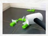
After the adhesive has set, you can remove the LEV TEC wedges and clips easily with a rubber mallet on the walls and by mallet or your foot on the floor.
