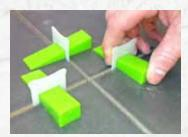
Using your thumb push the LEV TEC wedge with the right amount of pressure required to create the perfect finish.
