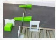
Set the adjacent tile firmly into the adhesive. Butt the tile against the LEV TEC clip giving the 1.5mm joint (if a larger joint is required spacers can be used, or set the required joint size).
