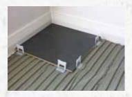
Spread your tile adhesive and lay the tile. Place LEV TEC clips underneath the tile slightly back from the edge.
